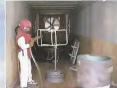
Remove old finish by sandblasting.
