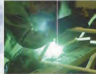
Straighten and re-weld frames.
